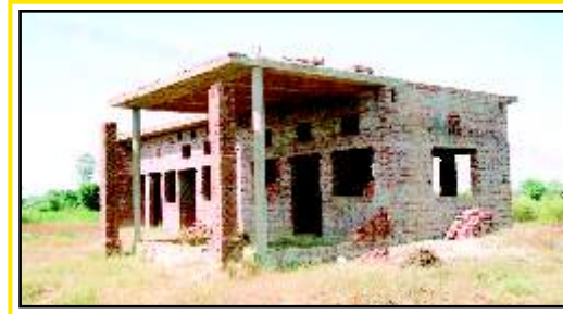
Nirmal Kutia – Vill. Bhattiwal-Kalan, Distt. Sangrur (Under construction)
