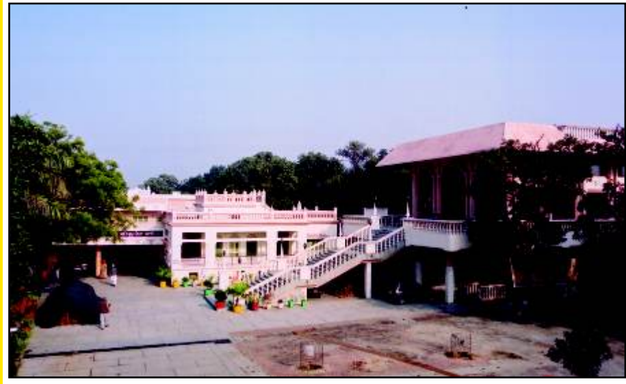
A view of Sri Darbar Sahib Bhawan, Satsang Hall and Ashram building.
